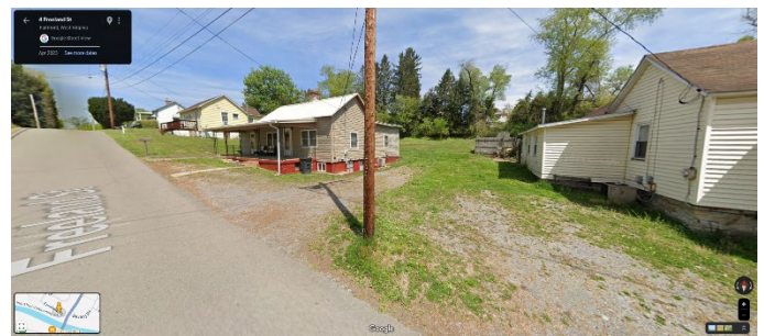
Figure 4 - Screenshot of Google Street View of Gravel Driveway Area Before Unauthorized Garage was Placed
