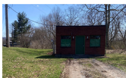
Glendale Lift Station
