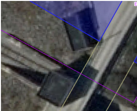
Log Stop Building and Flood control water outlet Building control by Water Dept.
