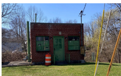
Cherokee Lift Station
