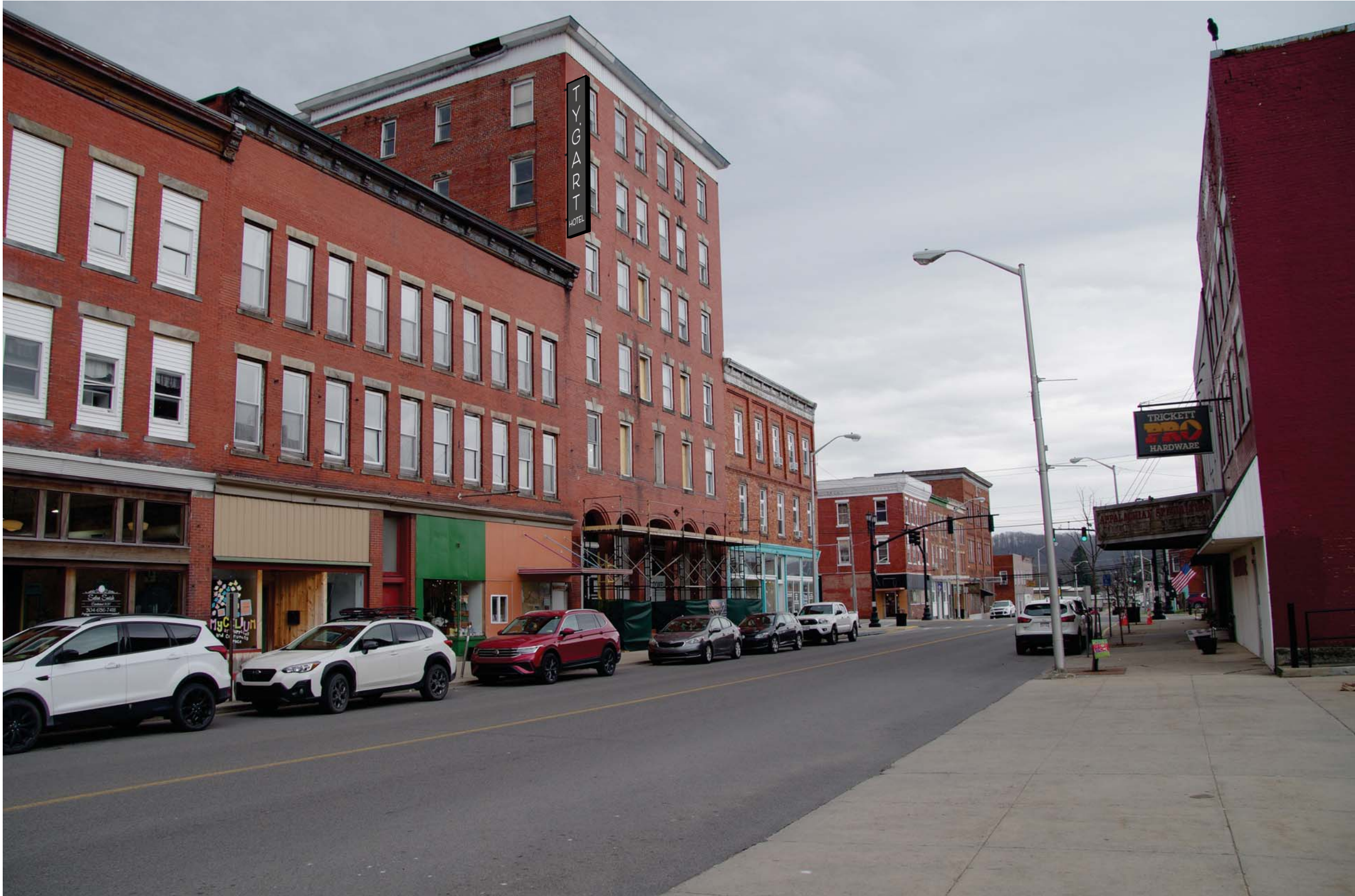
Corner Location Discussed at Site Meeting
